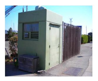
The Locust Street pump station was built in 1953 and is located approximately mid way along the District's interceptor sewer. It pumps sewage from Sausalito, Marin City and Tamalpais Community Services District to the gravity sewer on Bridgeway, upstream of the Main St. pump station. In wet weather some flows are diverted to Scotty's pump station, which pumps the sewage directly into the Locust Street pump station force main.
